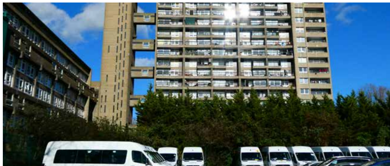
Figure 6.4: Existing car park, former care home site.
