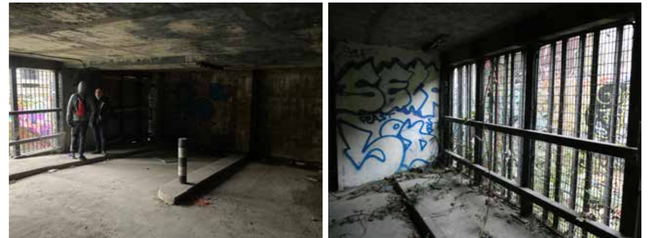
Figure 5.11: Inside Trellick's podium
